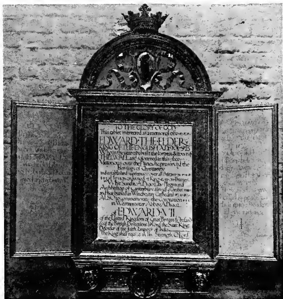
FIG. 124.—EDWARD THE ELDER. DEAL WITH WALNUT DOORS. INSCRIPTION PAINTED ON MIDDLE PANEL AND IN BURNISHED GILT GESSO ON WINGS. THELWALL CHURCH. F. C. Eden. 1907.
